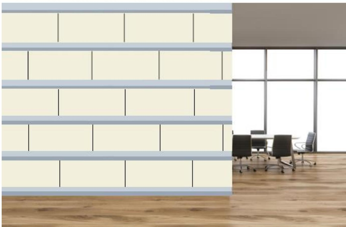
Then, mineral wool with thickness of 50 mm is put into the gaps between the racks.
