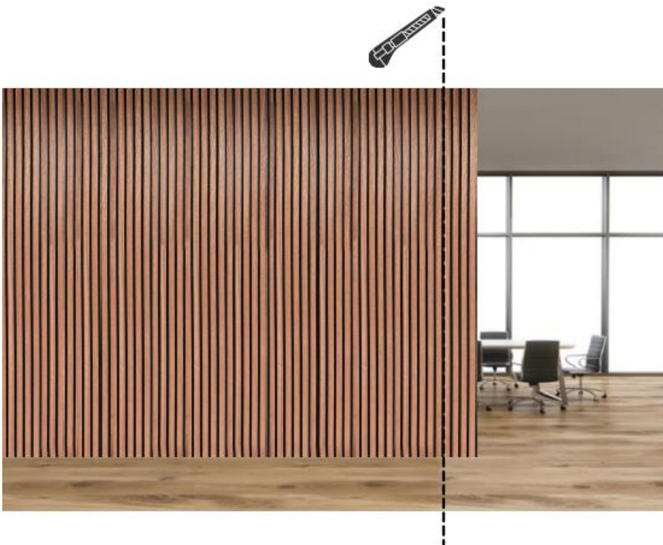
If there is less space left at the end of the wall than the width of the panel, we recommend cutting the panel along the rack with a knife to the width you need.
